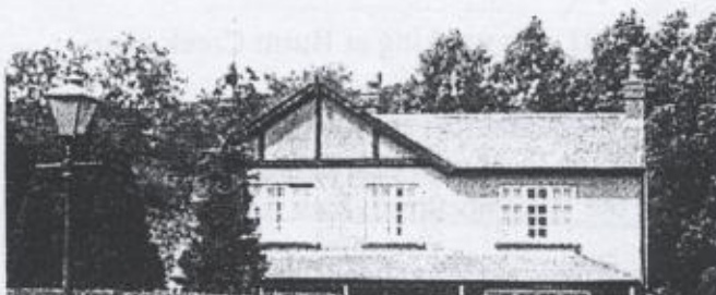
Manager's residence Darley Dale
